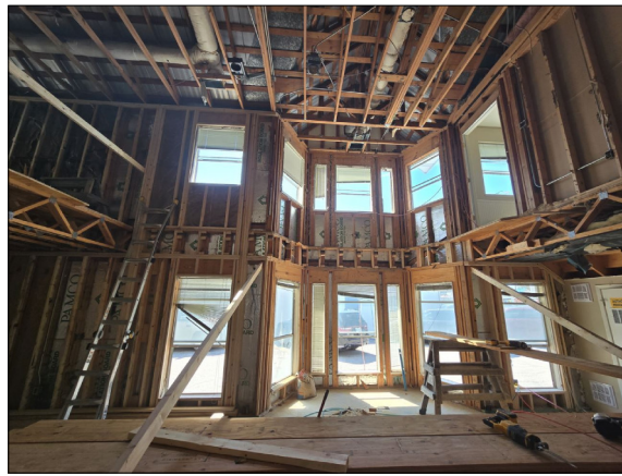
SECOND FLOOR BEING REMOVED
