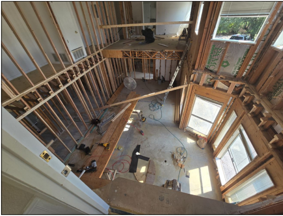
SECOND FLOOR BEING REMOVED
